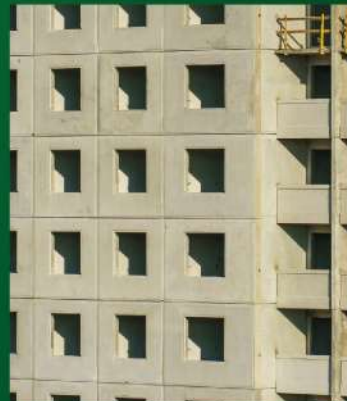
In an industry-first practice, Damp Proofing done to ensure no seepage or dampness.
